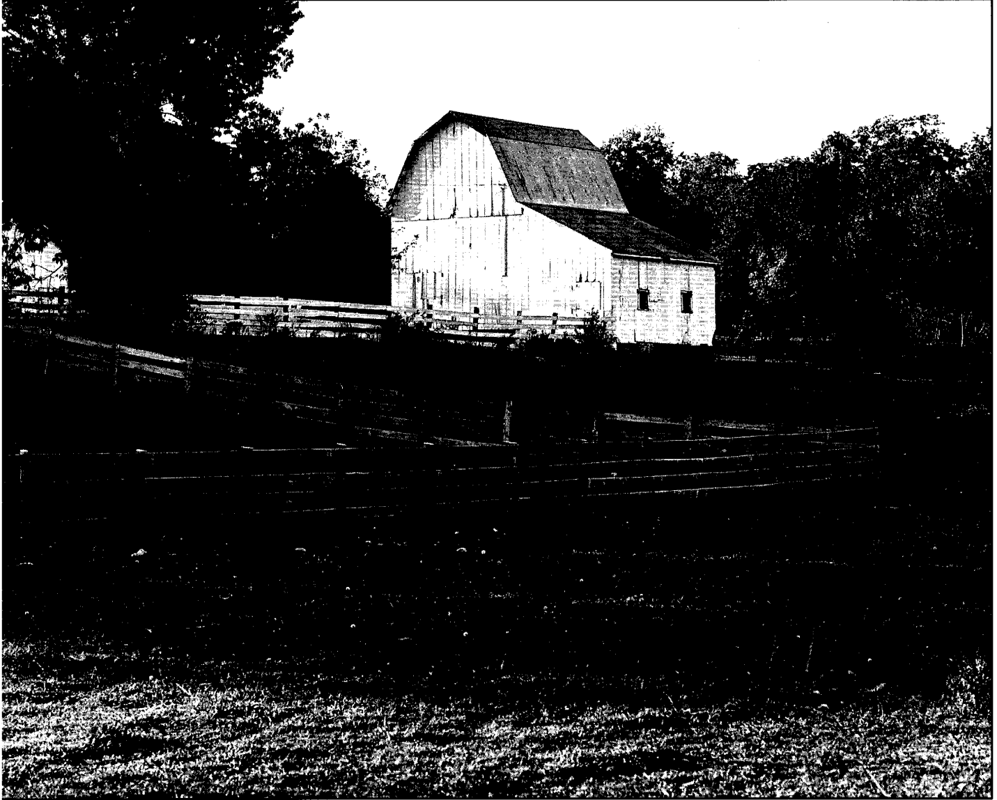
Small Gambrel Roof Barn with Side Addition, Charleston, Illinois
